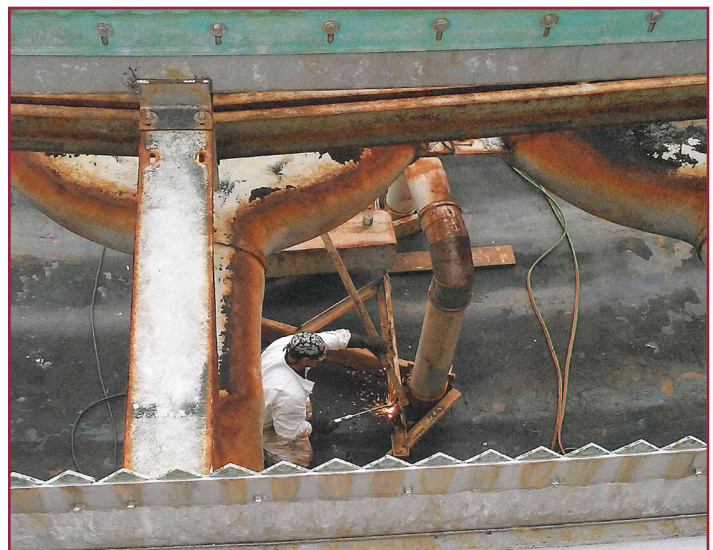
Repairs being made on Tank B-25 at W. Jefferson Avenue Wastewater Treatment Plant
