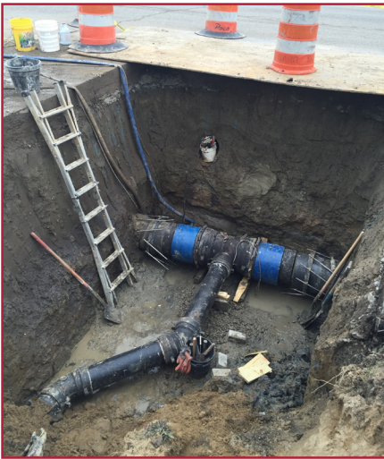
Replacement of Water Main Piping
